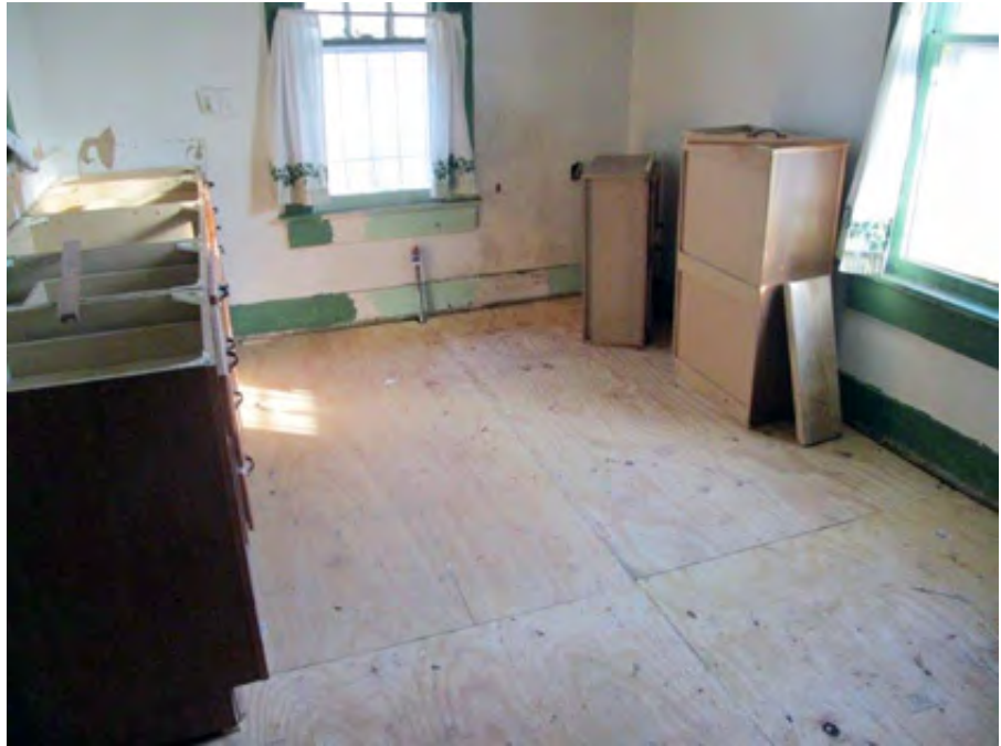
Kitchen floor repair 3
