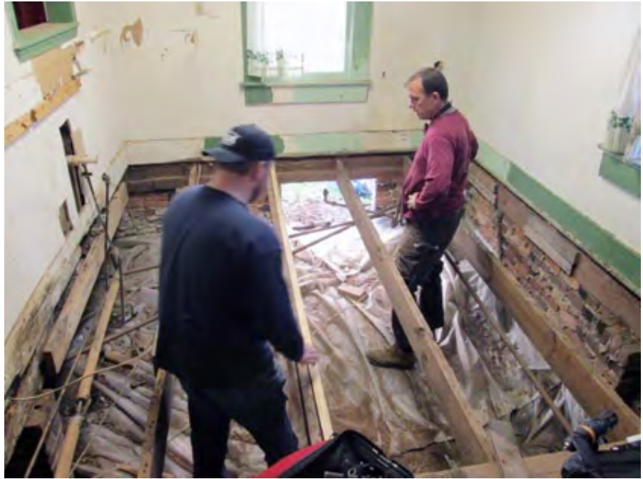
Kitchen floor repair 1
