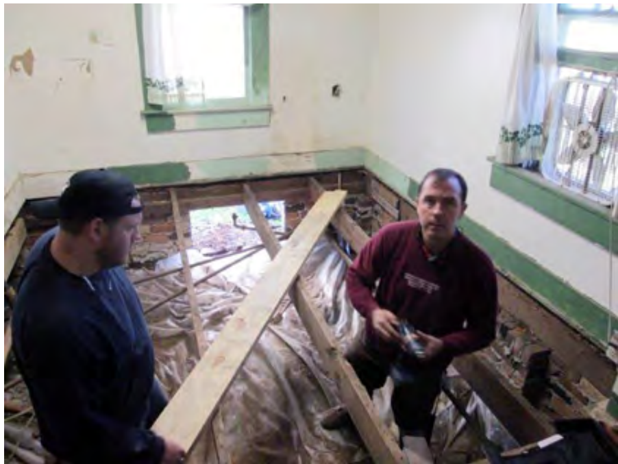
Kitchen floor repair 2
